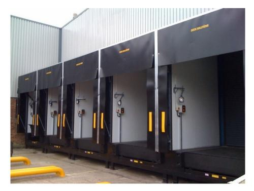
Dock Solutions Load houses can of course be disassembled and relocated if required meaning that your investment can go with you should you move, they also protect your main building from vehicle impact damage which can prove to be extremely expensive.
