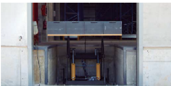
Single scissor lift with segmented lips
